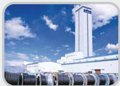
• Hwaseong 2 nd Plant
